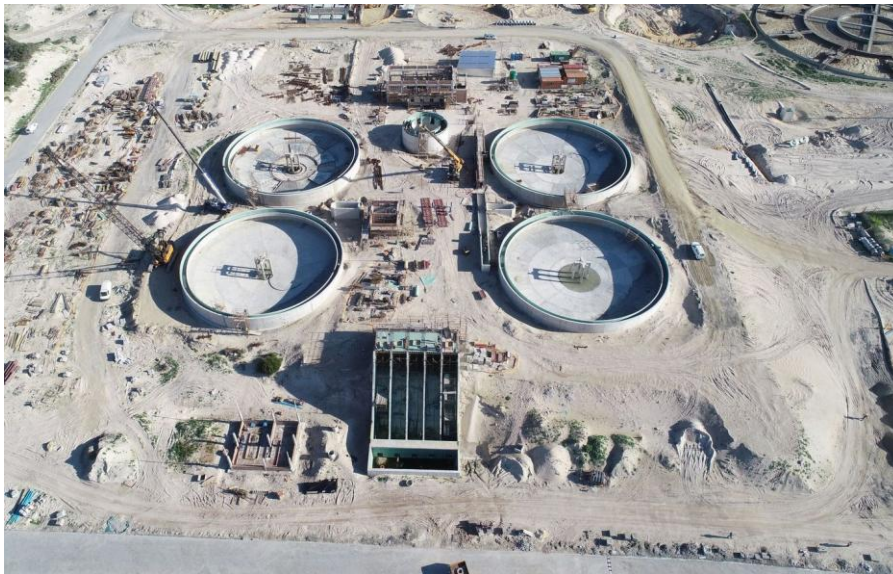
Above Picture - Zandvliet Waste Water Treatment Works
